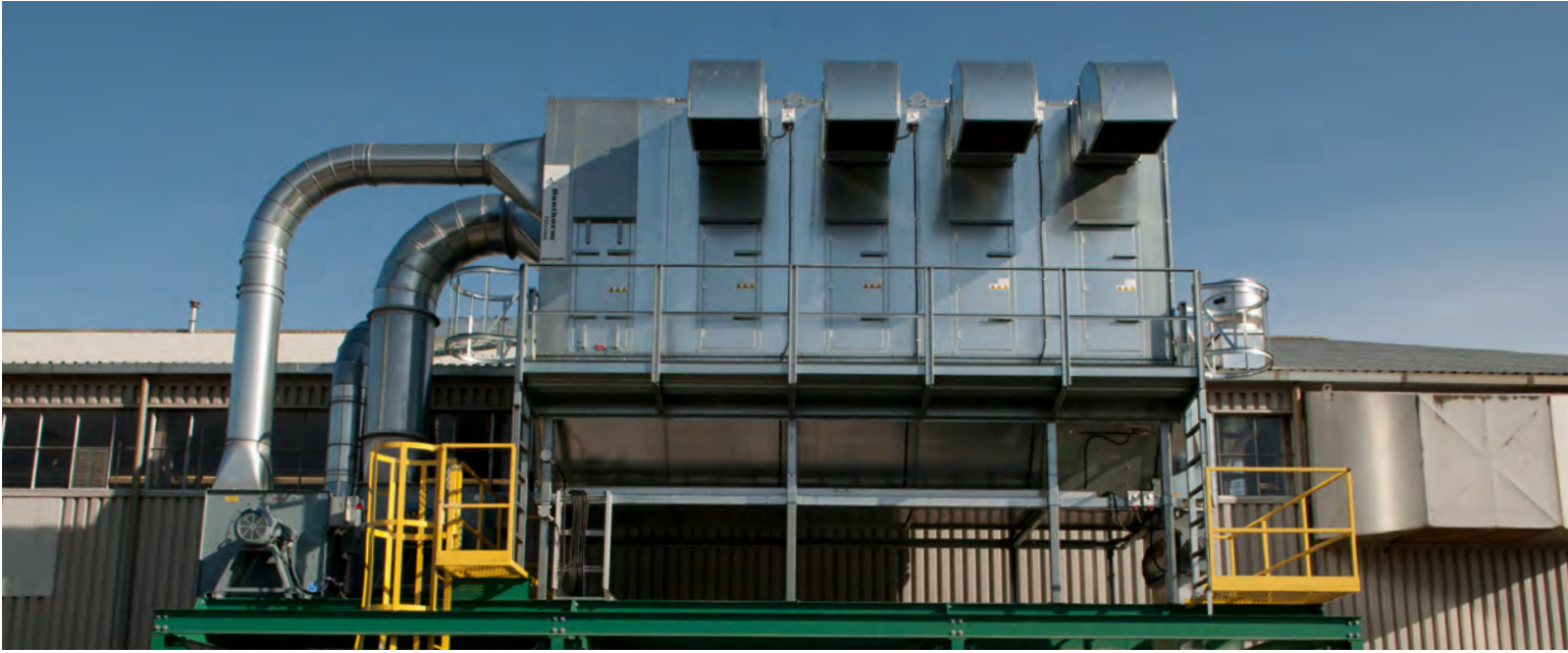
Part of the wood fuel preparation and storage system that feeds into the 300 kW biomass boiler.
