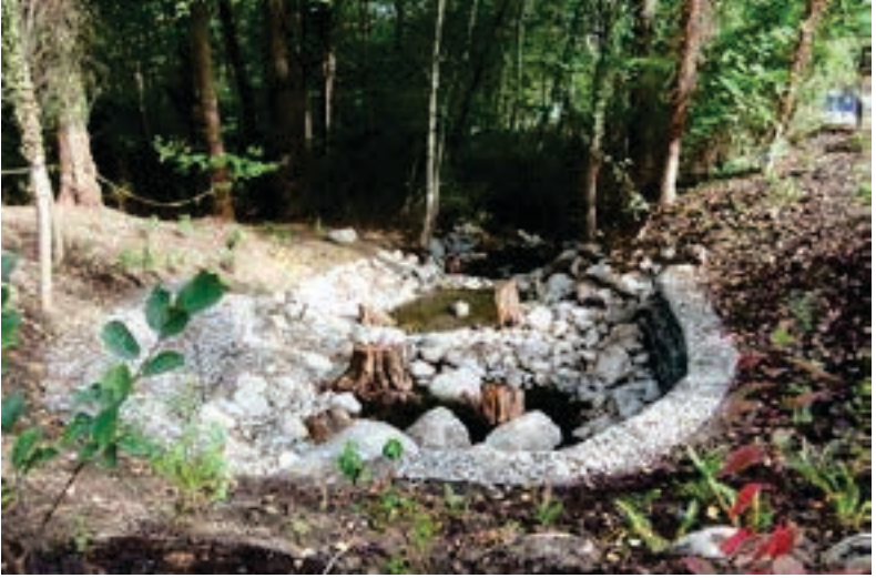
Guichon Creek restoration, associated with small-scale landscape characteristics (gabions and stone supports) re-established native plant communities, and restored natural systems (Blue and Green Design)
