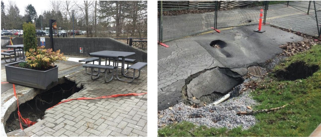
SE16 sinkhole (left) and Kyle Street sinkhole (right)
