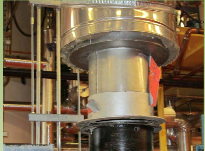
Cleaver Brooks boiler flue gases exhaust
