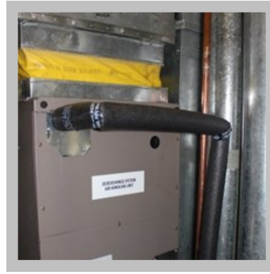
Geoexchange System Air Handling Unit
