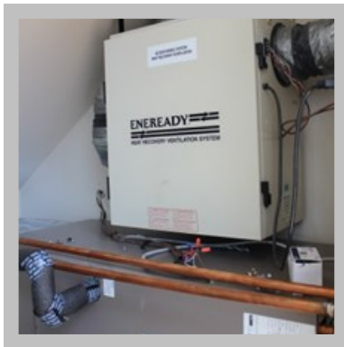
Geoexchange System Heat Recovery Ventilation
