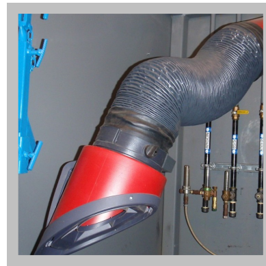
Local air extraction using telescoping arm
