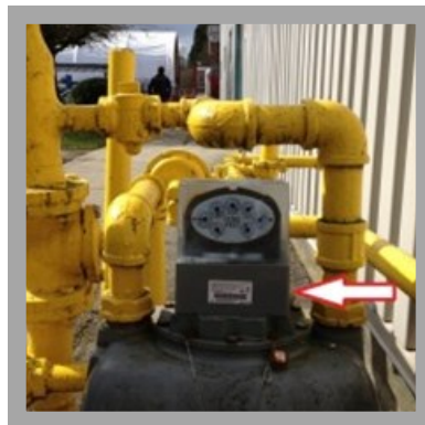
Itron ERT 100G Natural Gas Module
