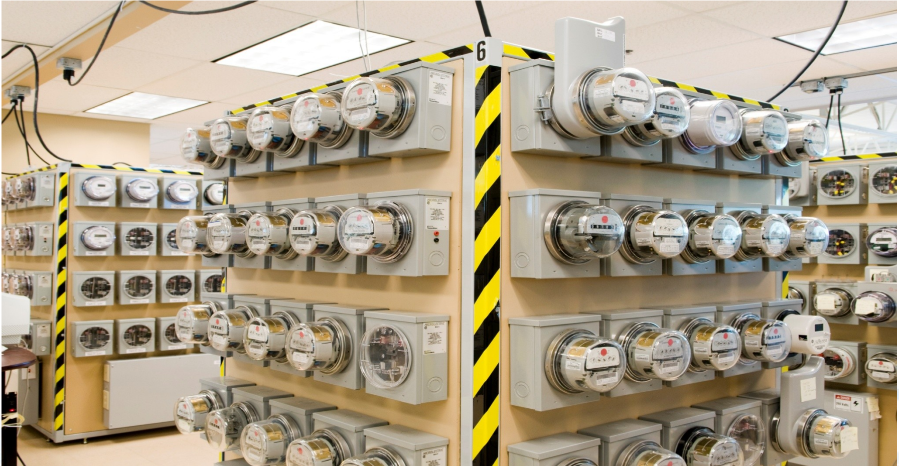
Smart Metering Farm
