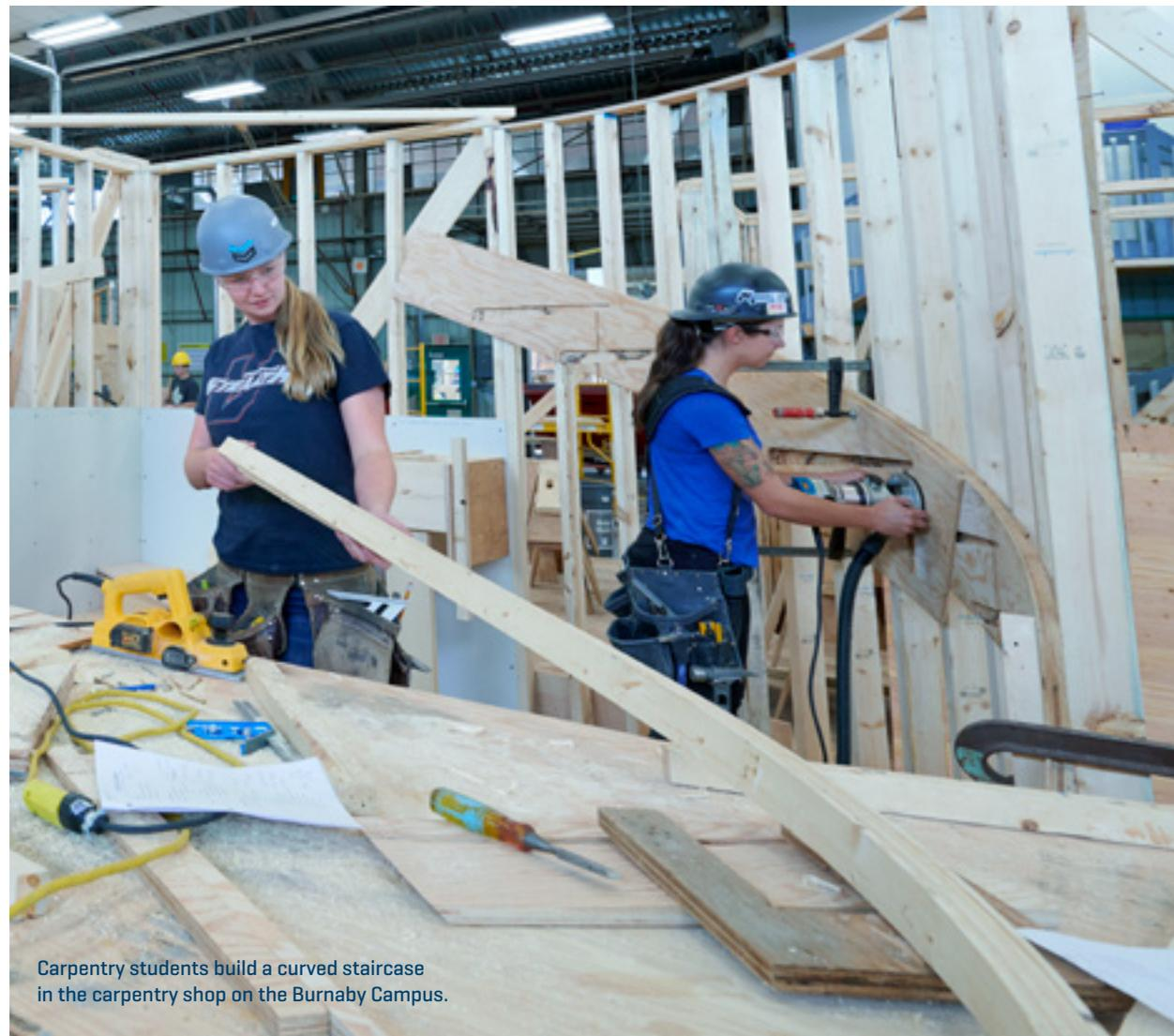
Carpentry students build a curved staircase in the carpentry shop on the Burnaby Campus.
