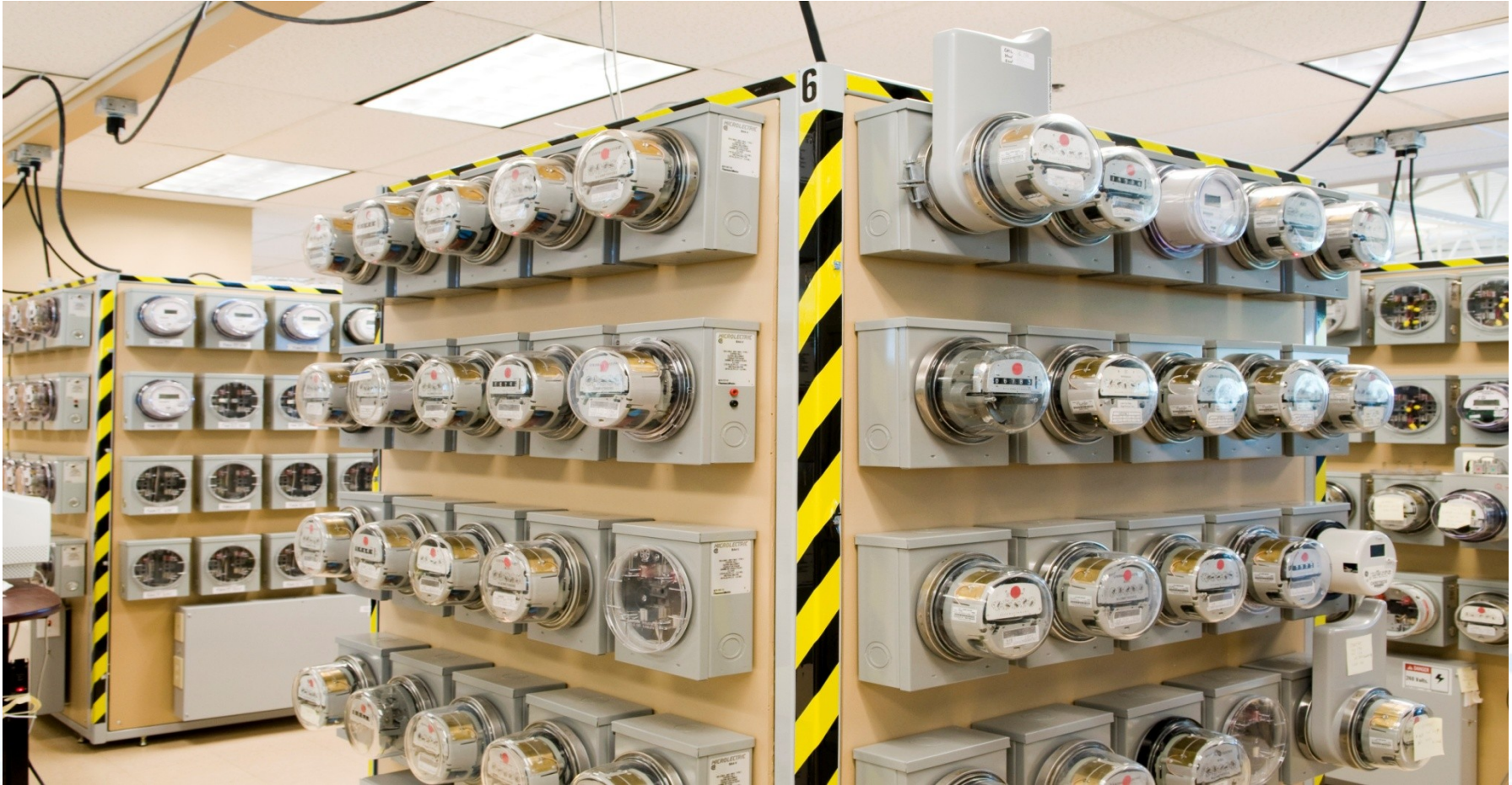
Typical Metering Farm
